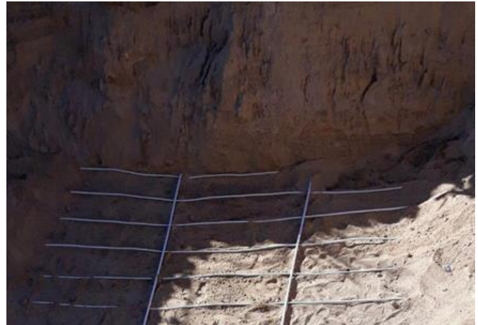
Fig. 3 MLCP pipes buried on depth 3 m.
